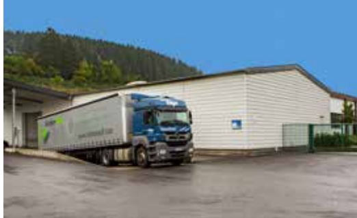
Figure top left: Warehouse in Kückelheim, Germany
